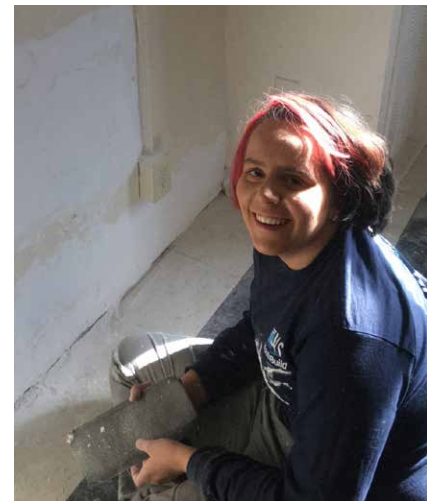
A YouthBuild student builds her drywall repair skills.
